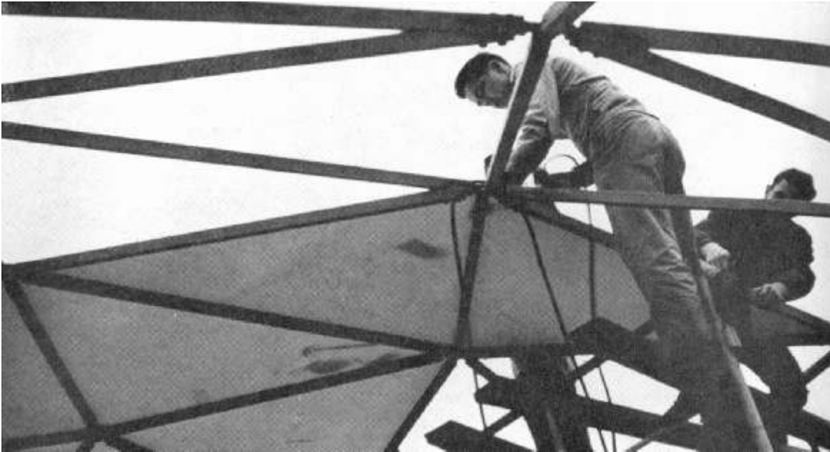
Dome of wood strut and canvas membrane construction, put up in 1957 by the design students
