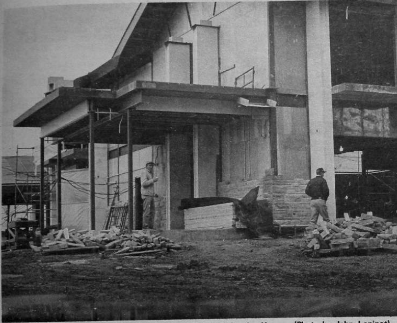
Construction continues on the controversial $975,698 University House. (Photo by John Lopinot)
