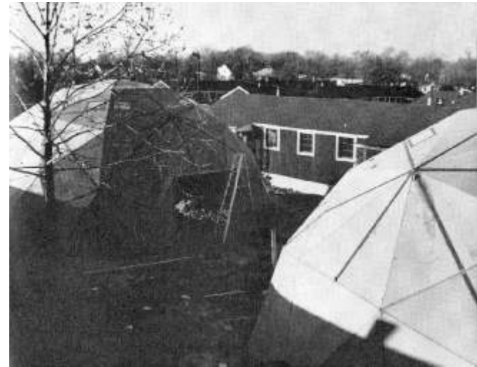
A general view of the department with two workshop domes in the foreground
